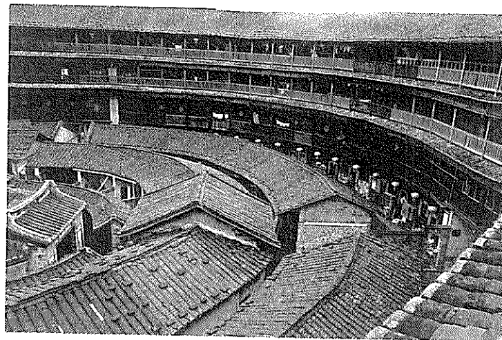
Thousands of toulou , clan dwellings of the Hakka, still dot the mountains of Fujian. Made from rammed earth mixed with rice stalks, they had no windows on lower floors as a defensive measure.
